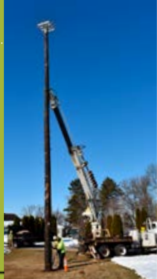
Installing an osprey nest in Stoughton, Wis.
