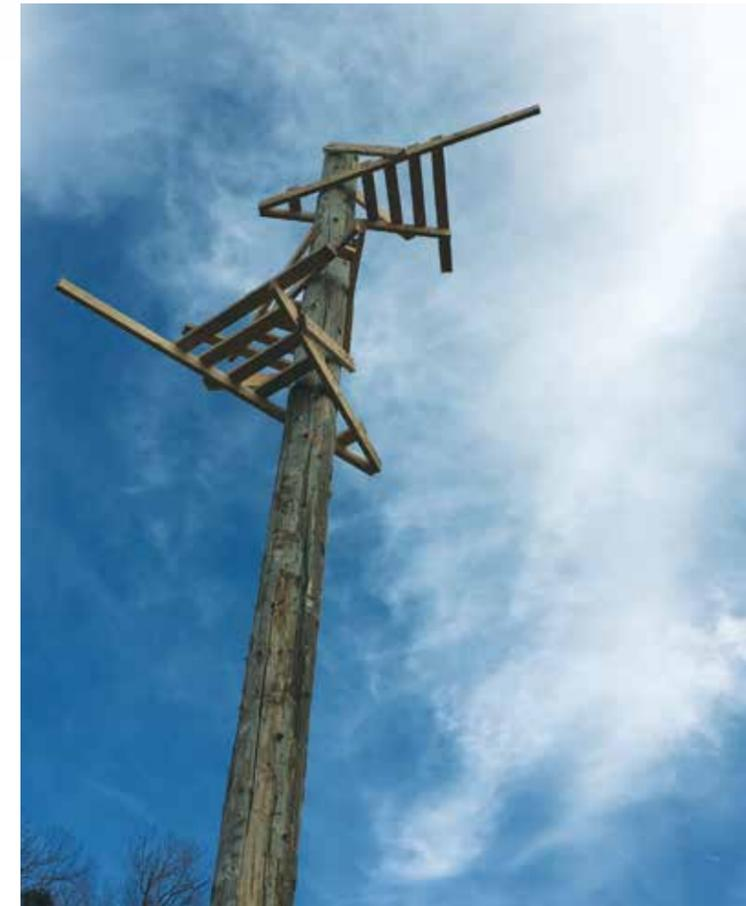
Each pole ATC installs for great blue herons contains three nesting platforms, which are installed at different angles to mirror the offset tree branches the birds prefer.
