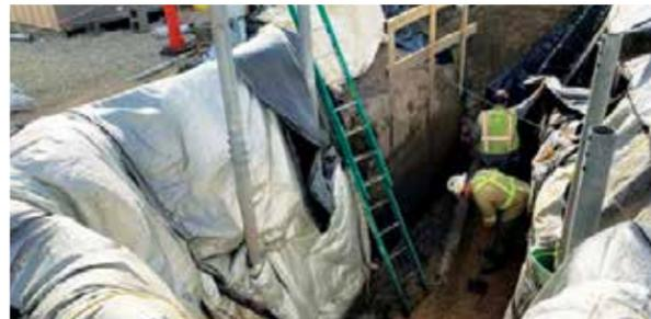
Rather than installing a shoring box, ATC froze the ground around an excavation area to improve safety and limit contamination.
