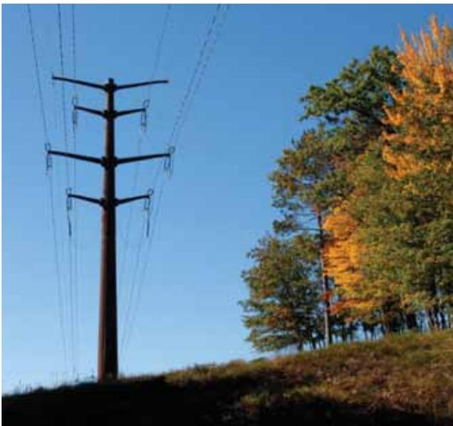
ATC's program takes into account tree and vegetation growth rates, line sagging and blowing, maintenance cycles, extreme weather conditions, and the potential for arcing electricity—a dangerous situation that occurs when electricity “jumps” from the wires to another source that can conduct electricity. When all of these factors are combined, the safe clearances between trees and power lines are larger than past practices or than many property owners believe are necessary.
