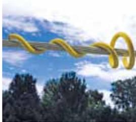
Bird flight diverters increase visibility of transmission lines.
