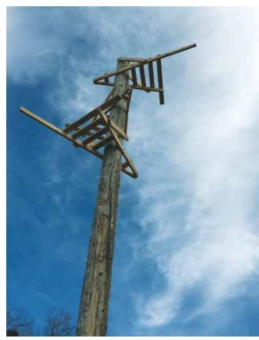
Each pole ATC installs for great blue herons contains three nesting platforms, which are installed at different angles to mirror the offset tree branches the birds prefer.
