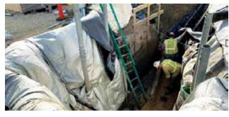
Rather than installing a shoring box, ATC froze the ground around an excavation area to improve safety and limit contamination.
