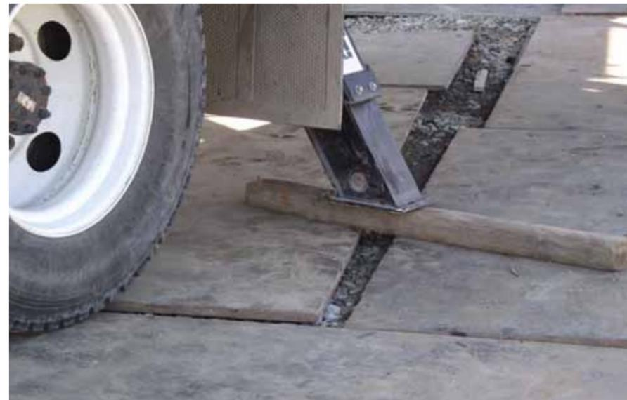
Road plating equalizes the weight over underground transmission lines.
