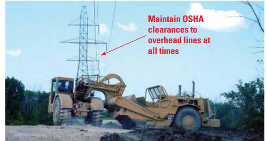
Wires move with wind and sag when warm. On a cold day, a lightly loaded line may hang 35 feet above the ground. On a hot day, or if the line is carrying a large amount of electricity, it may sag to only 25 feet above ground.
