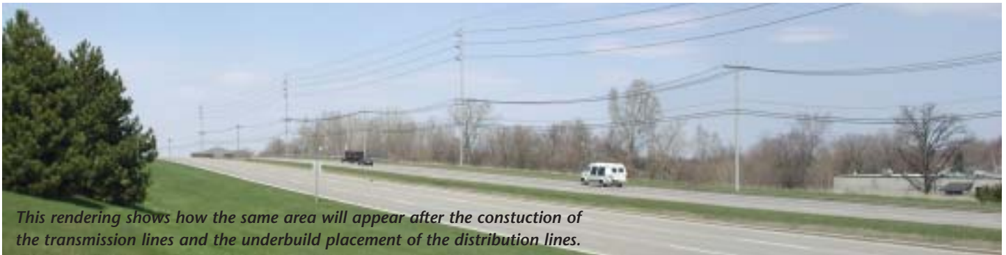
Looking northeast along Hwy. 164 at I94, the existing distribution lines are shown.
