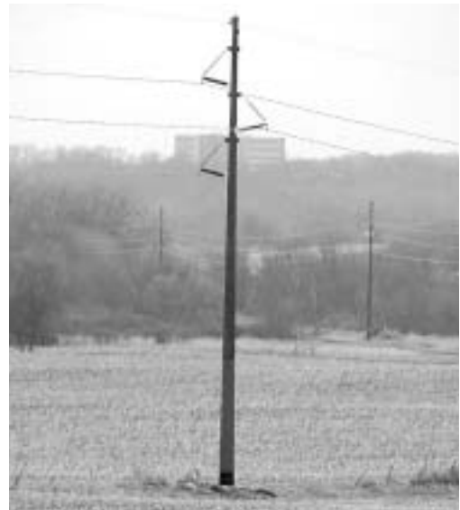
Single-pole weathering steel will be constructed on existing right-of-way.
