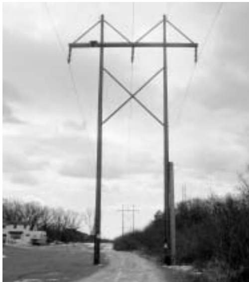
Existing H-frame structures like the one shown above will be removed.
