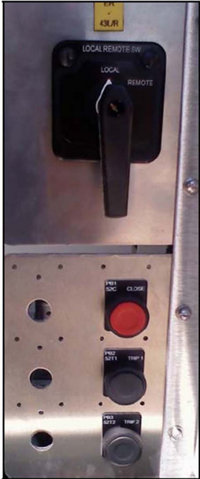
a. Controls in 138 kV Breaker Cabinet
