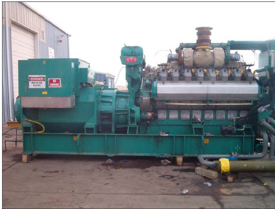
3.2.8 MVA New Age Cummins-Wartsila diesel generator unit.
