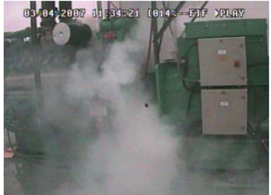
Figure 9. Smoke and pieces of generator coupling being ejected.
