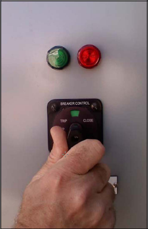
b. Controls in Relay House
