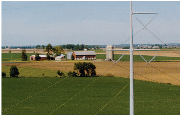
Single steel poles for 345-kilovolt transmission lines are typically 110 to 120 feet tall.
