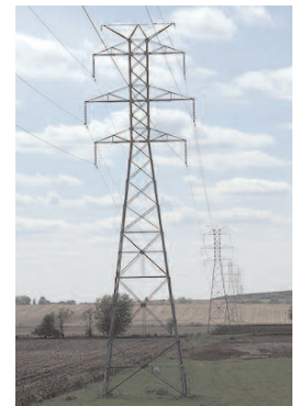
Lattice towers are generally not used in new construction.
