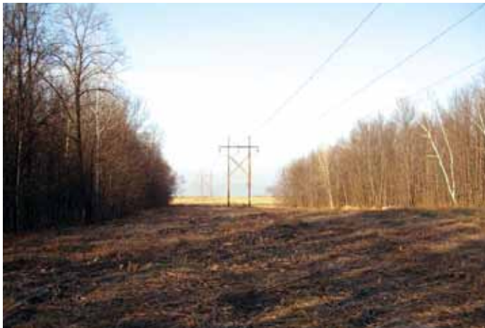
Photo of a right-of-way shortly after clearing work was completed.
