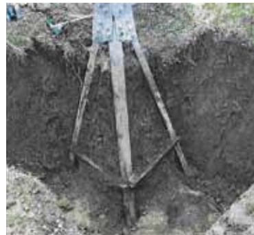
Buried transmission structure anchor
