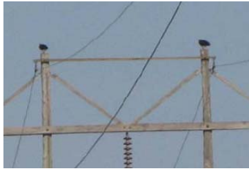
A pair of osprey sit atop a former h-frame structure (3/2007).
